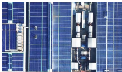
► Microgrid Power-Computing Upgrade Jiangxi | 2.8MWp PV + 5.4MWh ESS
